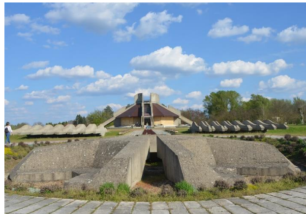
Figure 11 - Memorial Museum of the Battle of Batina on the Danube near Bezdan is a masterpiece of monumental modernist architecture in Sombor Region (Author: A. Grujičić, 2021).
