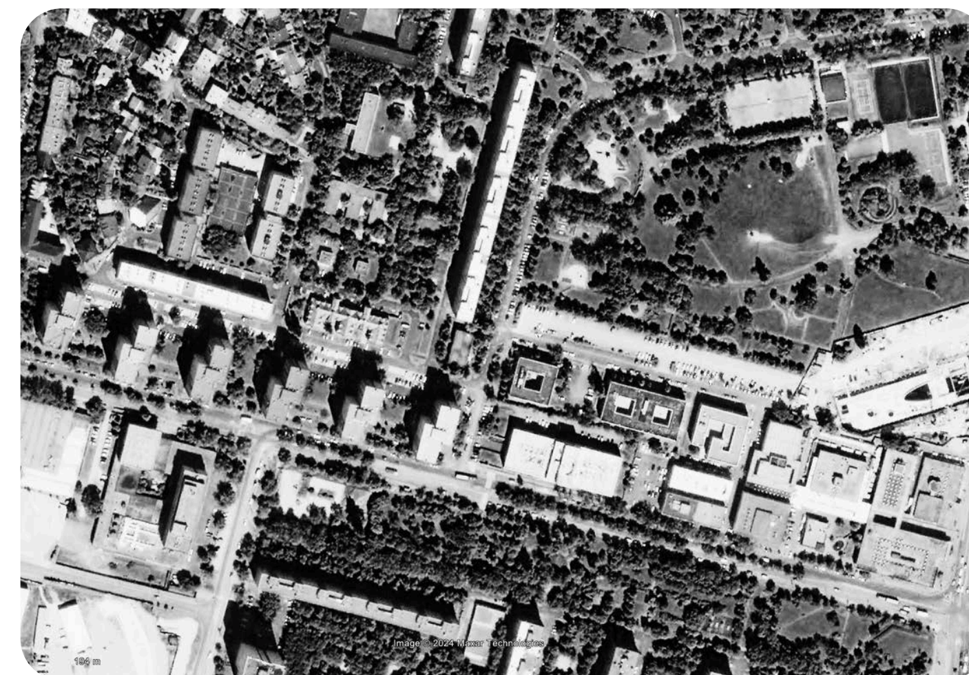
2007 Started construction of Bikás Park M4 station
