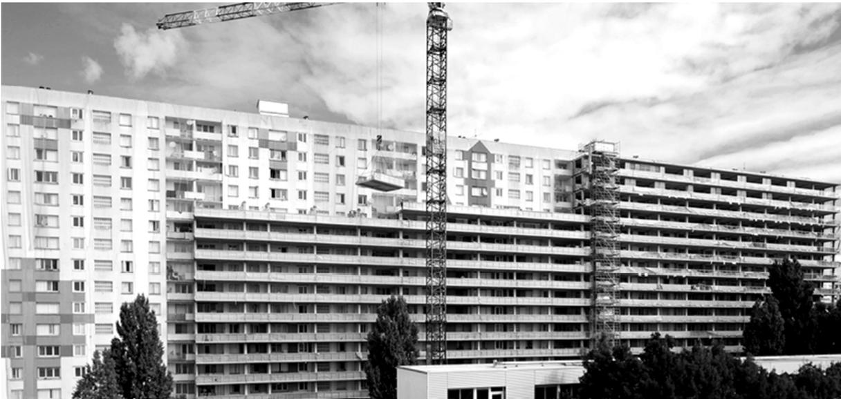
*Figure 7. Transformation (modernization) of housing blocks in Bordeaux, France, according to the Lacaton Vassal architecture office design. Instead of fulfilling contemporary thermo-insulation needs by just adding the Styrofoam to façade, Lacaton and Vassal added “new skin” to the building, which also provided residents with additional living space.*
