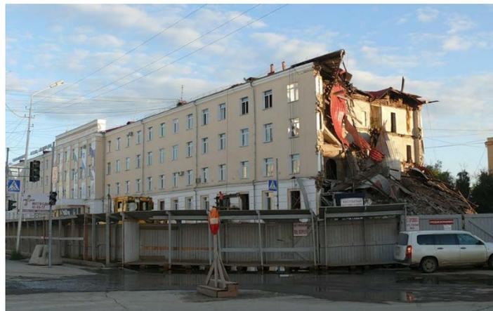
Figure 4. Building damaged by permafrost melting. Source: Euromaidan Press, 2016.
