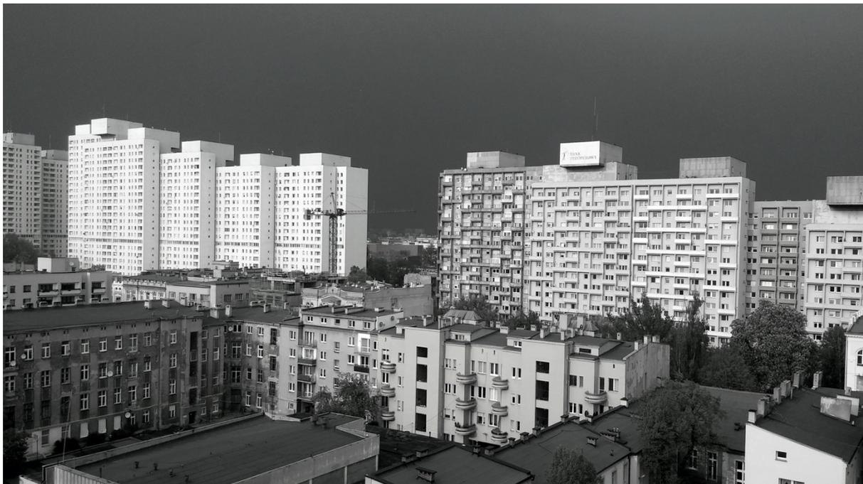
*Figure 2. Housing Estate called Manhattan, located in Lodz city center. On the photograph the “modernization” of the blocks is visible, block on the right side is just partially covered with layer of styro-foam as thermo-insulation, while blocks on the left side are completely “modernized”. With this action the original façade is demolished, and the tectonics of the elevation disrupted.*
