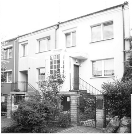
House complex in Kwiska Street, Wrocław, examples of house modernizations, 2017. Source: Author
