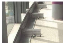
HALFEN Curtain Wall Brackets fitted to the top of a floor slab using HALFEN HTA Anchor Channels
