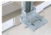
Curtain wall connection installed to the top of a floor slab using a HALFEN HTA Anchor Channel
