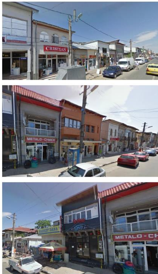
Figure 22 Protected architectural assembly in Giurgiu, cf. official list of monuments and sites, http://www.cultura.ro/lista-monumentelor-istorice
